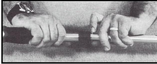
6. Wrap the cable around the pole leaving enough slack near the searchcoil to permit searchcoil adjustment. Note: Do not allow the cable to flop loosely over the searchcoil. Since the detector is sensitive enough to “see” the tiny wires in the cable, a floppy cable can cause false signals as the searchcoil senses the moving wires.
